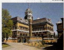
Bazalgette designed a system of underground sewers for the city. The splendour of the Abbey Mills Pumping Station expressed all that public Victorian society could not about the importance of sanitation.
